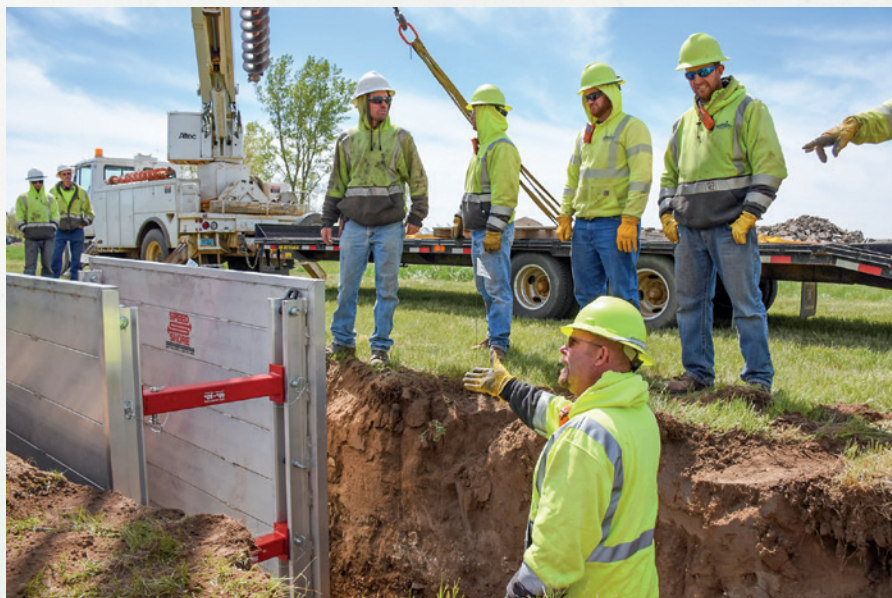
In the spring of 2017, Slope Electric Cooperative hosted trench box training with area cooperatives. Craig Turner (in trench), former line technician for Slope and current safety instructor for the alliance, served as one of two resident experts who provided guidance on assembly and use. A trench box is a steel or aluminum structure that is used to protect utility workers while performing their duties within a trench. Customarily constructed with sidewalls of varying thickness held apart by steel or aluminum spreaders, the box can withstand a collapse without buckling.
