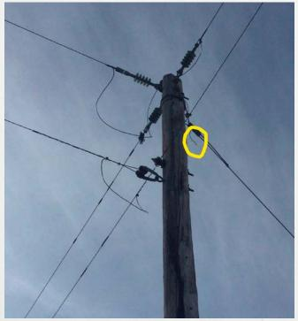
The yellow circle shows a broken ground wire; it was spotted on line patrol and corrected before the system became compromised and an outage occurred.
