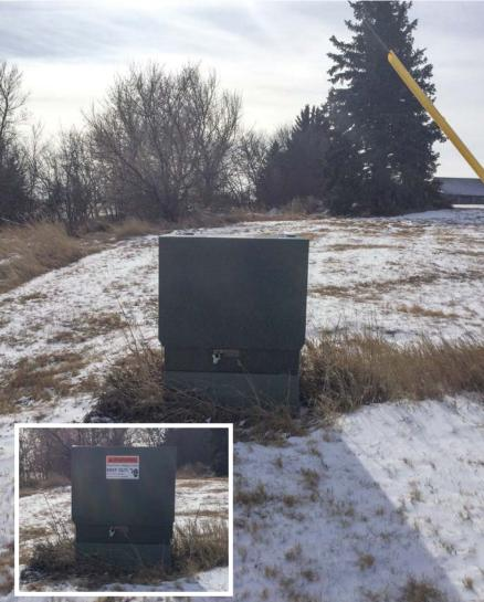
This photo shows how a strong North Dakota wind can deteriorate and remove cabinet signage over time. The missing safety reminder, spotted on line patrol, is quickly corrected (see inset) to remind the public of a possible danger. Always keep a safe distance from electrical infrastructure!
