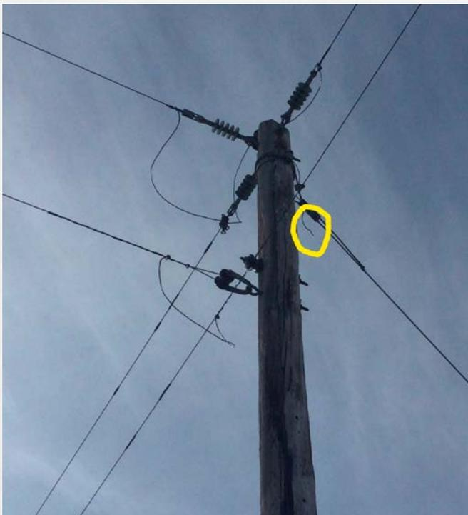
*The yellow circle shows a broken ground wire; it was spotted on line patrol and corrected before the system became compromised and an outage occurred.*
