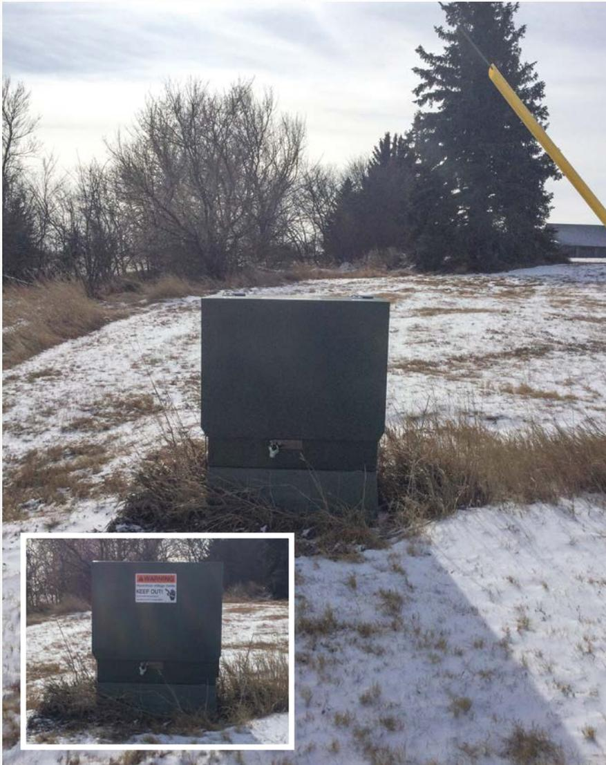
*This photo shows how a strong North Dakota wind can deteriorate and remove cabinet signage over time. The missing safety reminder, spotted on line patrol, is quickly corrected (see inset) to remind the public of a possible danger. Always keep a safe distance from electrical infrastructure!*
